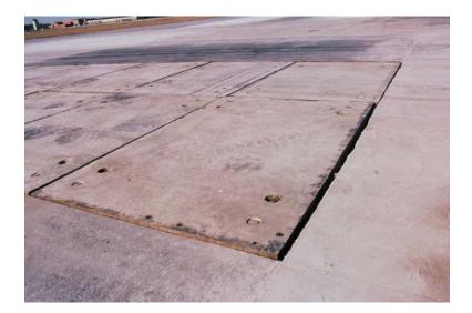
Figure 3-2. Temporary pre-cast panels at Savannah. (Photograph provided by Gary Skoog)
