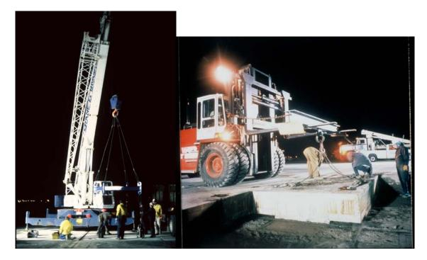
Figure 3-3. Larger crane used in Charleston (left) and smaller equipment used in Savannah (right) to place temporary pre-cast panels. (Photographs provided by Gary Skoog)
