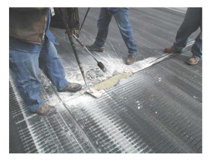
Figure 3-1. Placing patch material at Colorado Springs.
